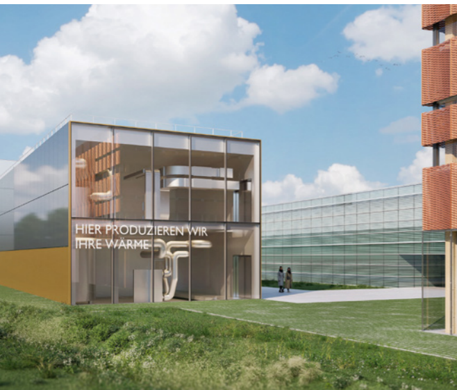
A processing facility located next to HLRS III will capture and distribute waste heat produced by HLRS supercomputers to the University of Stuttgart's district heating network.
